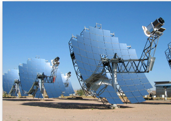
Dish Technology in California’s Mojave Desert Source: Stirling Energy Systems
